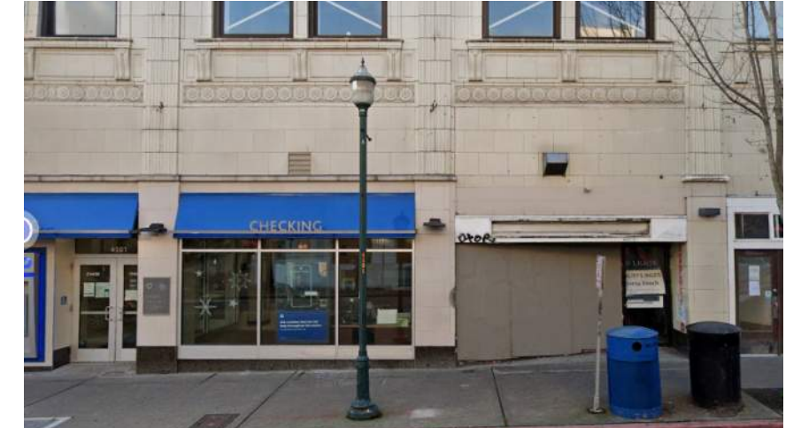
Ped light pole on The Ave
