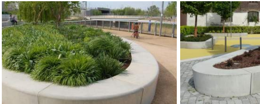
Raised precast concrete planters.
